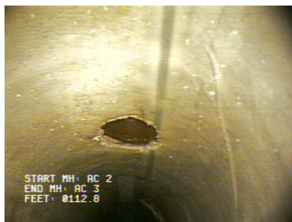
Sewer after lining
