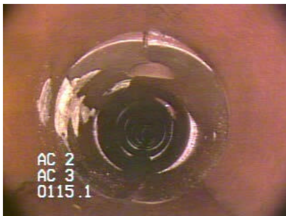
Sewer before lining
