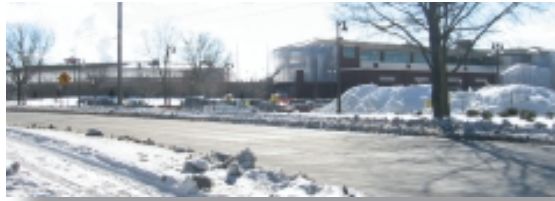
Dow Diamond Stadium Nears Completion
